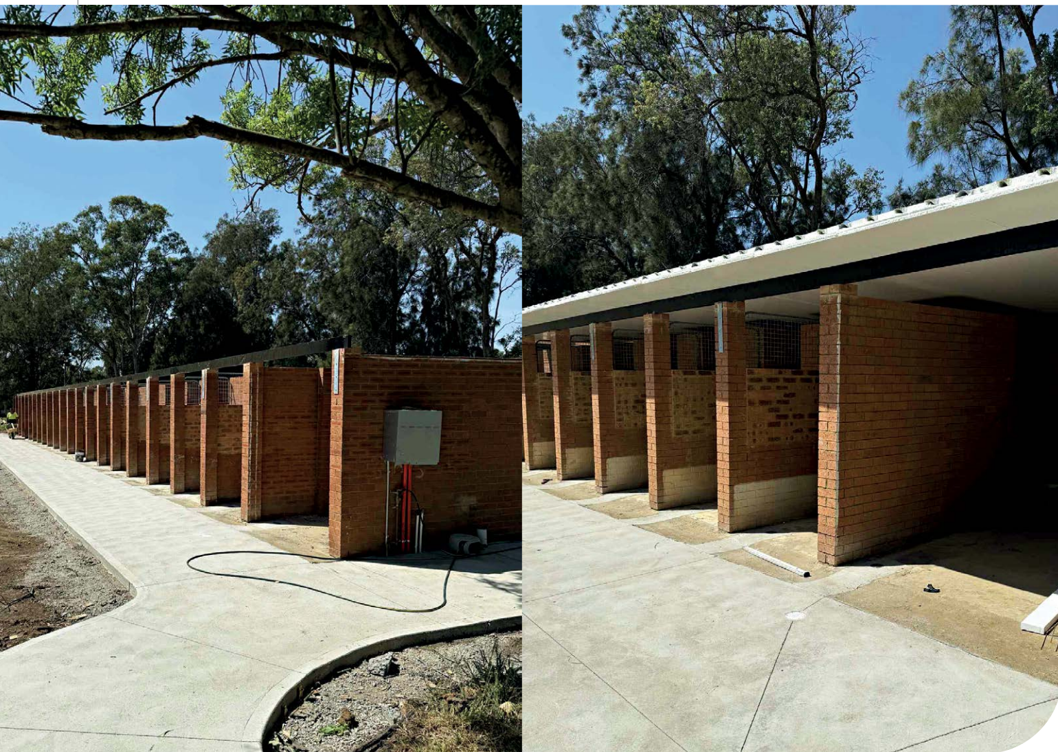
Progress underway on the refurbishment of the first two dog kennel rows at the new Precinct for Animal Welfare (PAW) in Rossmore.
